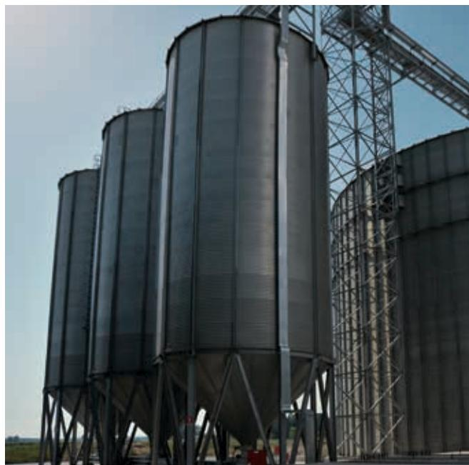
The thickness of the sheets and of the uprights is defined according to the model and the place of installation of the silo (the solicitations due to seism, wind and snow are also considered crucial elements). The calculation of the solicitations suffered is performed according to the norm DIN1055 part 6.
