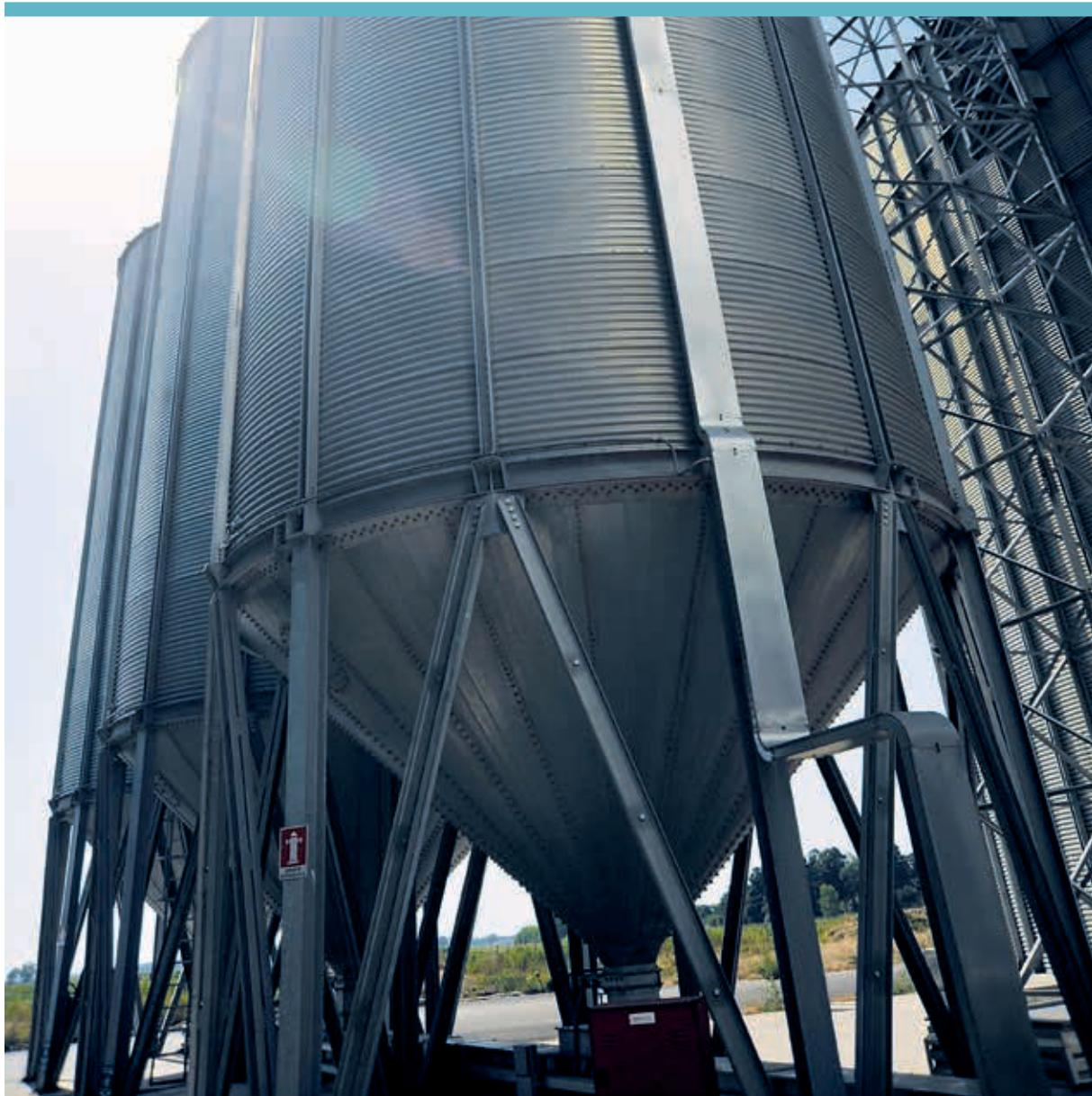
The metal hopper silos (TM serie) are used in the storages in which the complete unloading of the bins is needed without the usage of mechanical devices or operators' intervention. They are particularly indicated while storing cereals with difficulties in flowing both for the morphological conformation and for the high humidity level because the inferior hopper simplifies the gravity self-unloading.
