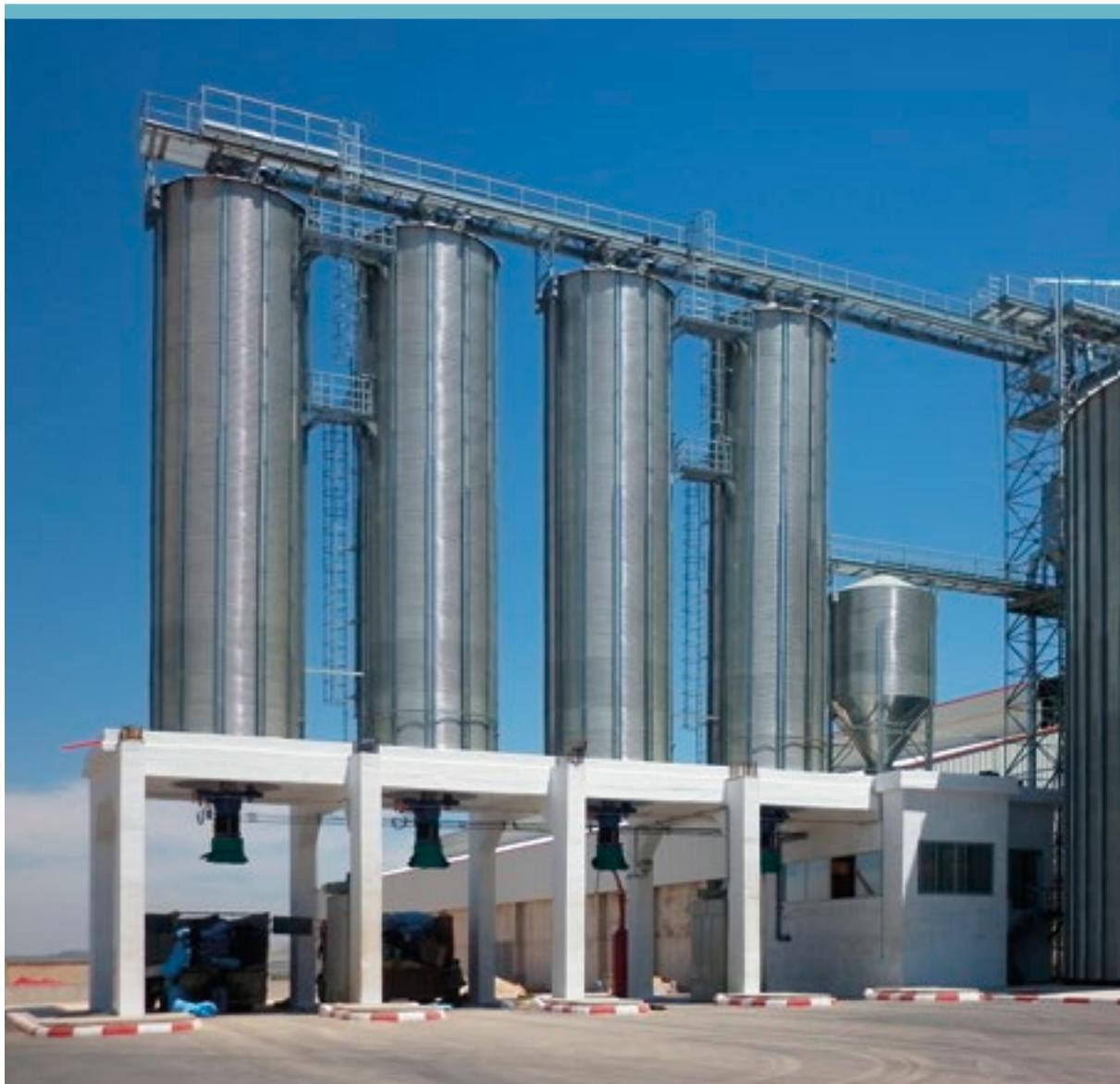
The quick loading silos (CR series) are used for loading means of transport such as trucks and trains.
