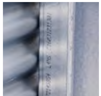
ENG. Every upright is marked on the back with the number of the coil from which it has been produced, the company identification code and the identification acronym
