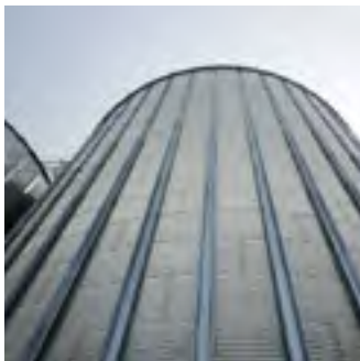
ENG. View of the silo cylinder and upright columns
